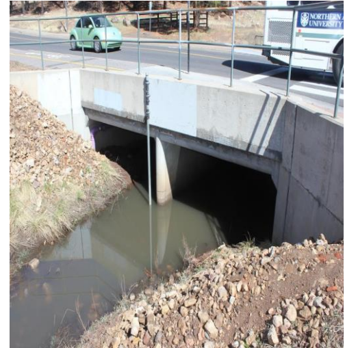
Figure 3: Culvert under South Knoles Drive
